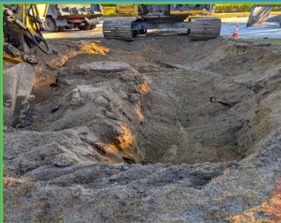
Longfellow Avenue main line replacement September 22, 2025
