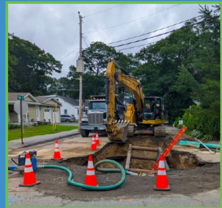
Page Street main line replacement July 8, 2025
